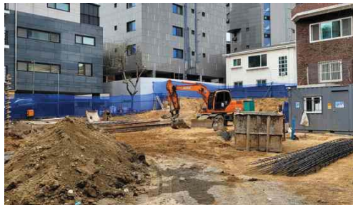
Photo. 1 Load Factor Analysis Based on Actual Construction Site
